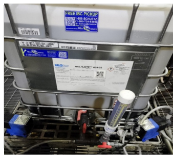
FIGURE 1: Nalco Water dosage point setup for the dispersant solution
